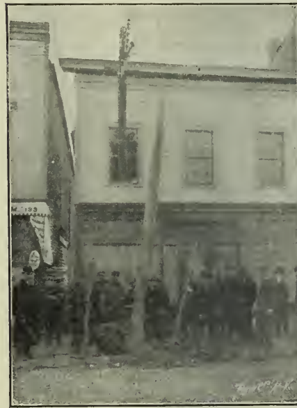
FIG. 2. TELEPHONE POLE CUT IN TWO BY PIECE OF BOILER
